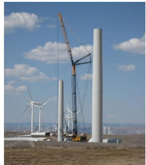
Wind turbine construction in Oregon.
