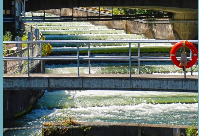
Fish ladder at the Bonneville Lock and Dam. Photo: U.S. Army Corps of Engineers, Portland Corps.
