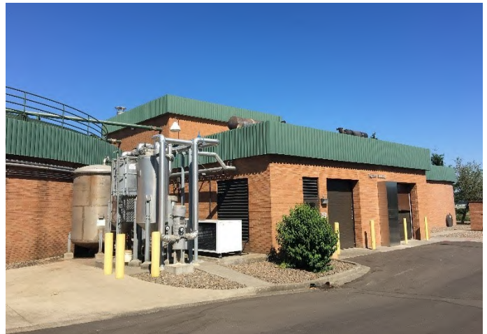
Gresham Wastewater Treatment Plant
