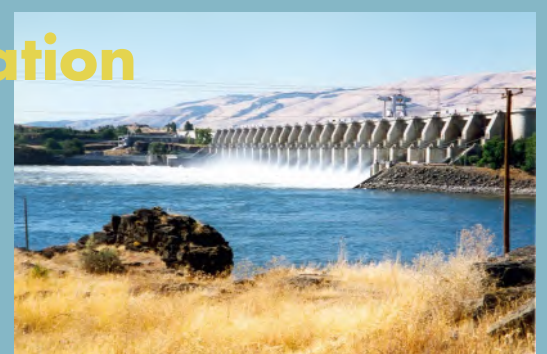
The Dalles Dam in the Columbia River Gorge produces up to 2,000 MW of power.
