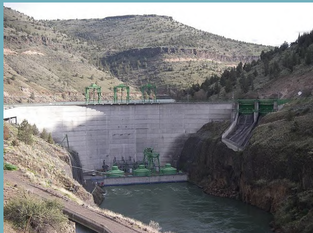
Pelton Round Butte Hydroelectric Dam Photo by U.S. Forest Service
