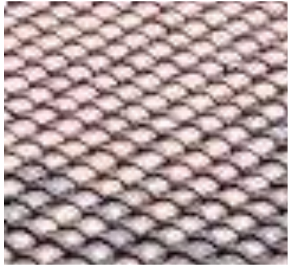
Red tile roof
