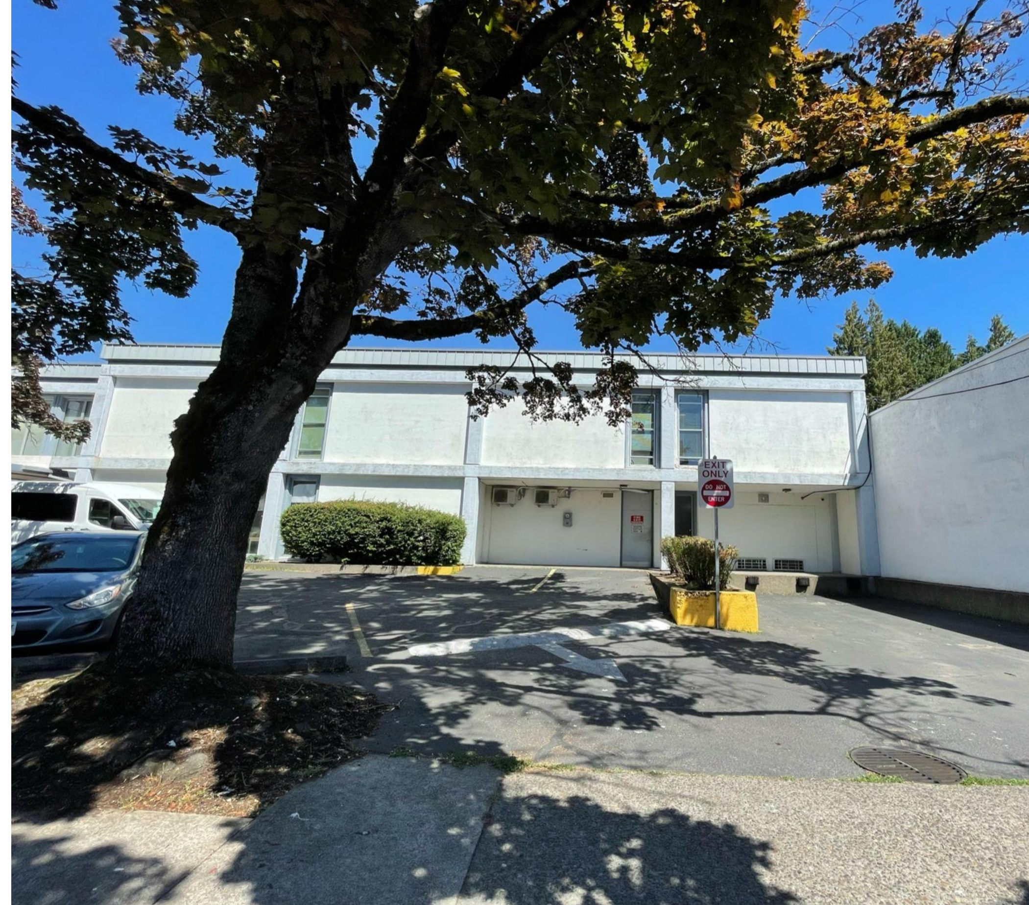
Loading dock & curb cut (1) at sidewalk Russell St.
