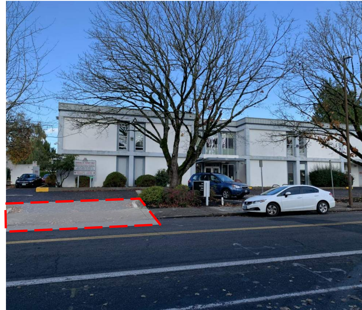
Curb cuts at Russell Street to be removed.
