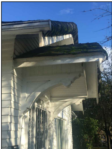
1.Porch Roof & Rolled Roof Edge
