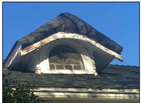
1. Attic Dormer & Rolled Roof Edge
