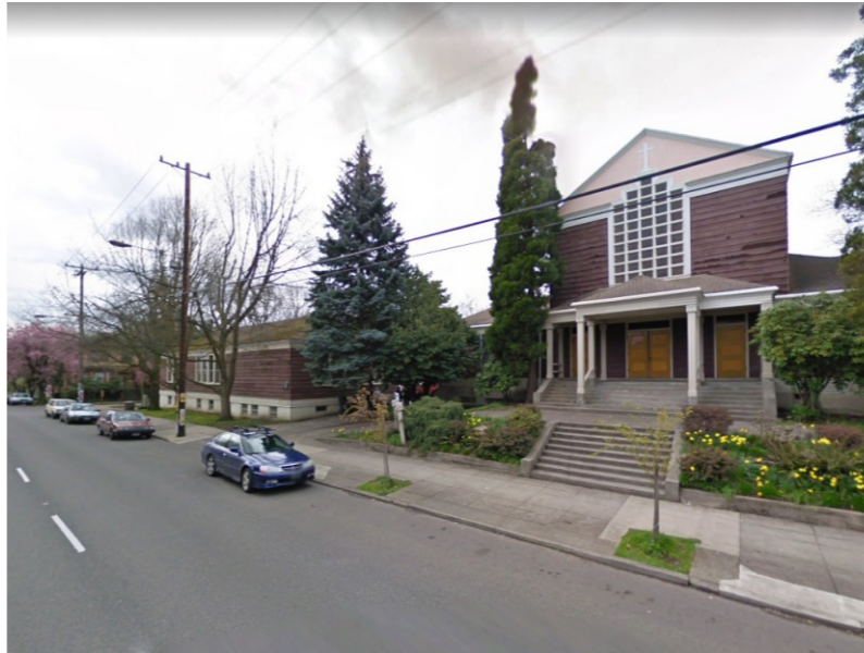
View of pedestrian connection to church
