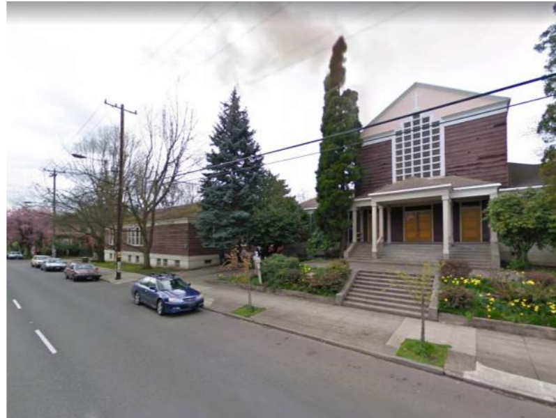
View of pedestrian connection to church
