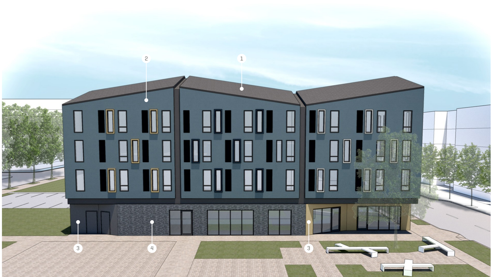
1. COMPOSITE SHINGLE ROOF
