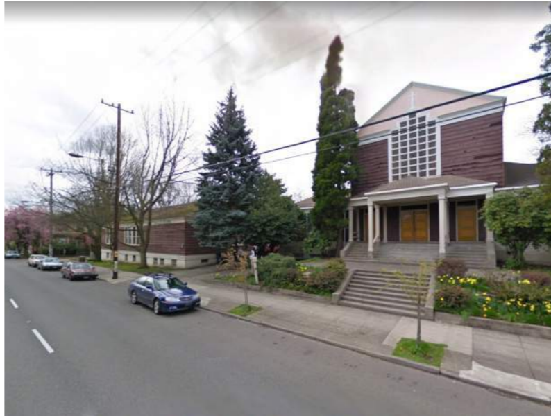
View of pedestrian connection to church
