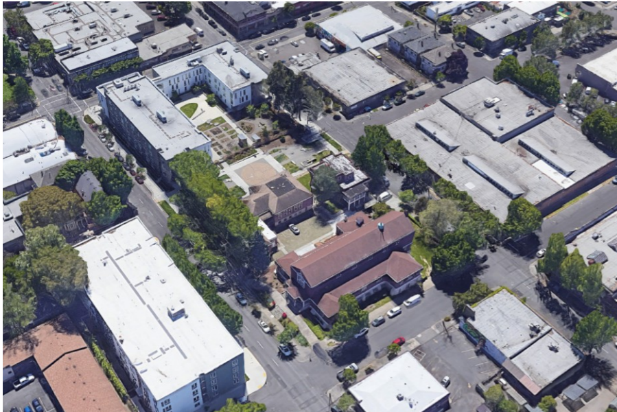
Aerial view from NE looking SW
