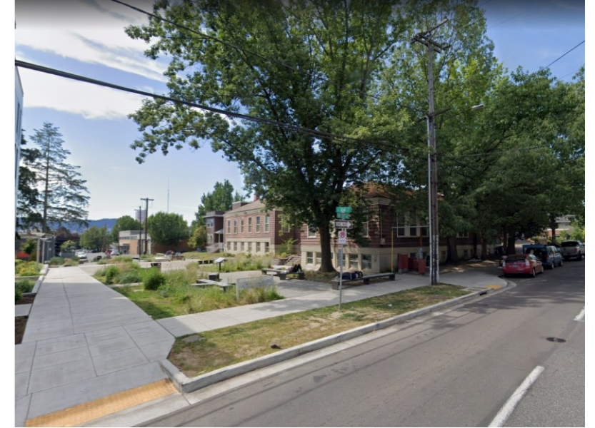
View of site from SE corner
