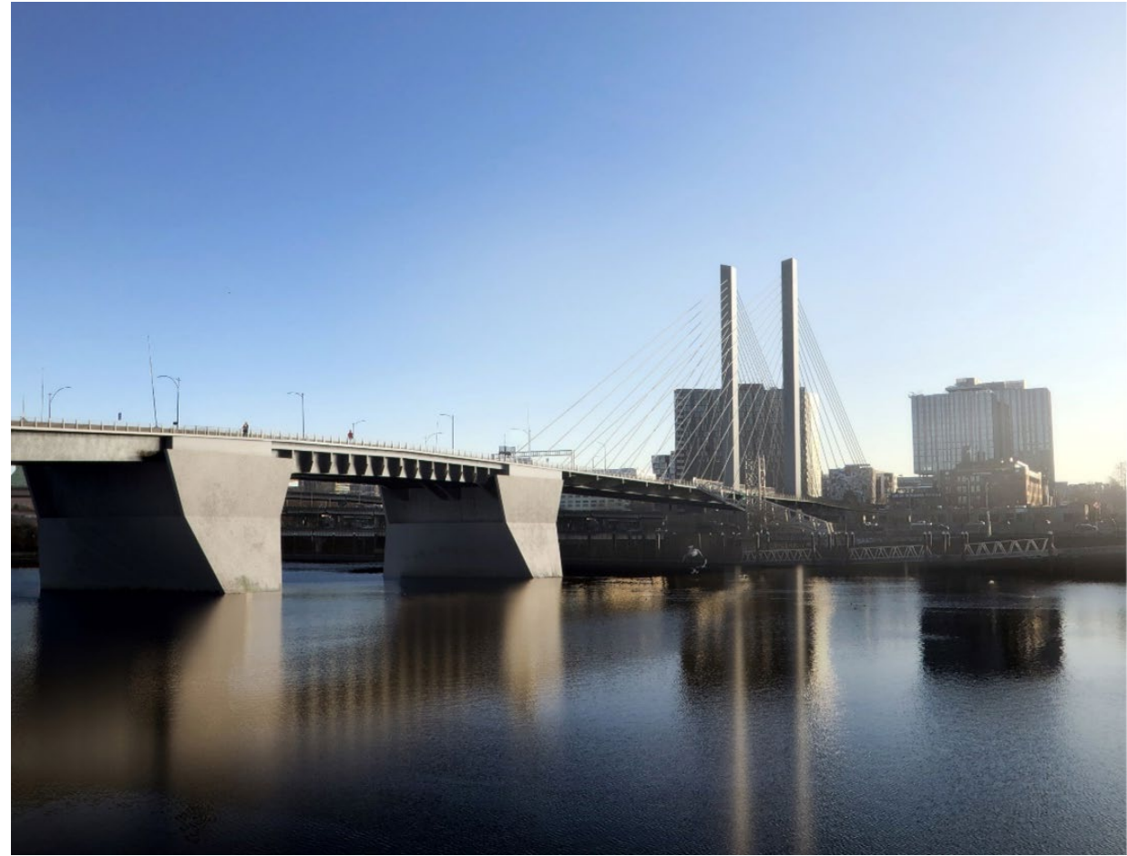
with Cable Supported
