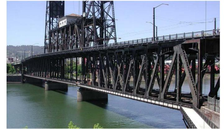
The Steel Bridge in Portland, combination rail-roadway-light rail lift bridge carries a multi-use trail adjacent to the lower lift deck.
