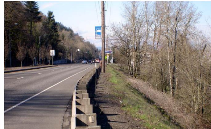
The existing ground falls away steeply. Some places include retaining walls very close to the guardrail and industrial facilities adjacent to the right-of-way.
