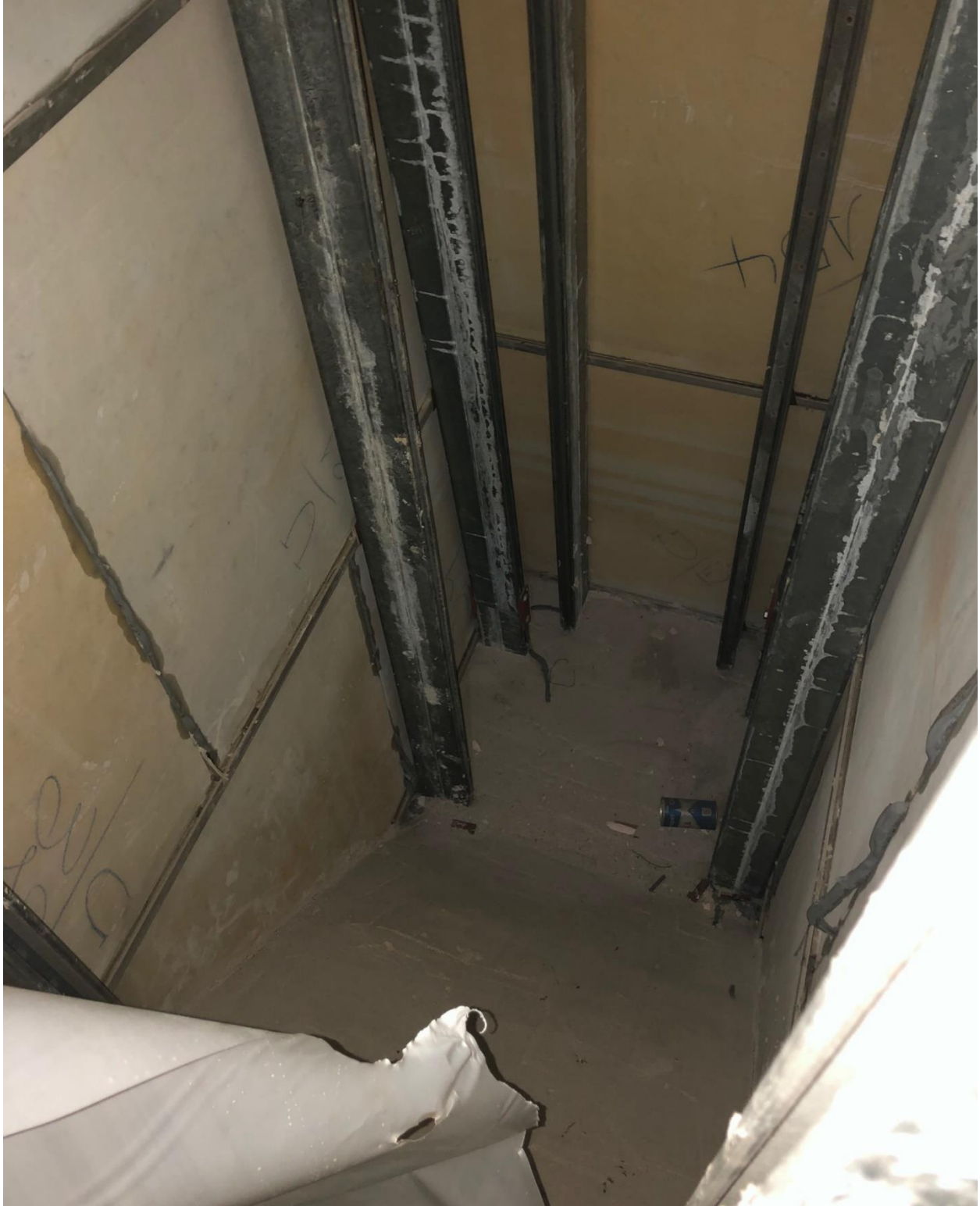
Photograph of the existing firestopping between levels 2 and 3, inside the stone column surrounds.
