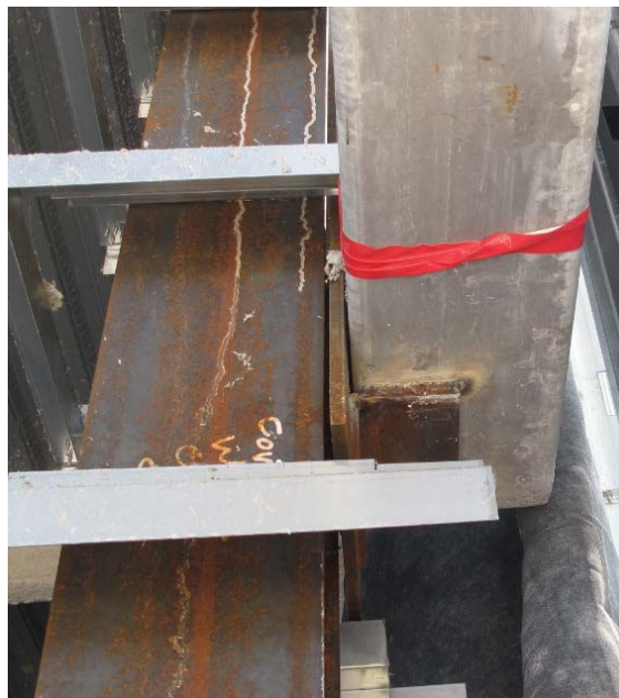
Outrigger to column attachment
