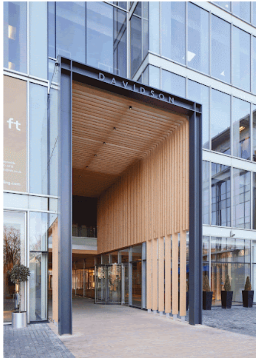
The Davidson House in Reading, UK has an elegant public passageway that links the north and south entrances. The space is well lit, has activating glass walls and has warm natural materials including a timber fin ceiling structure throughout.
