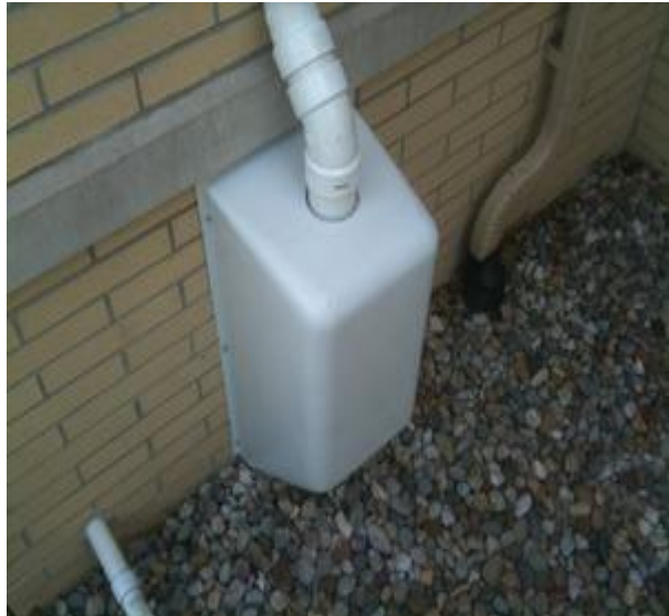
Radon Fan Cover Installation Example
