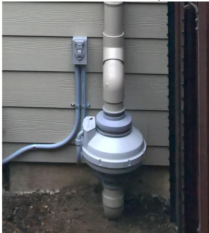
Exterior Mounted Radon Fan Example
