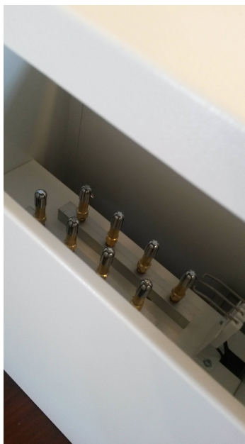
Photo Detail 6 – Gas burners on inside of unit
