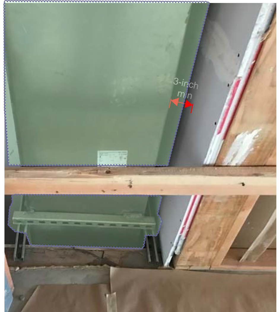
Vent Hood Duct - looking down
