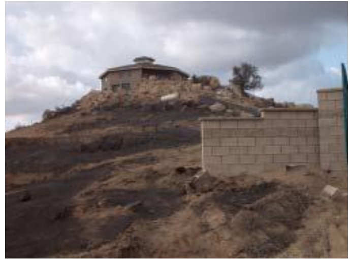
Wildfire blackened the landscape surrounding this residence, but the concrete masonry walls were unharmed. (Photo courtesy of Concrete Masonry Association of California/Nevada)
