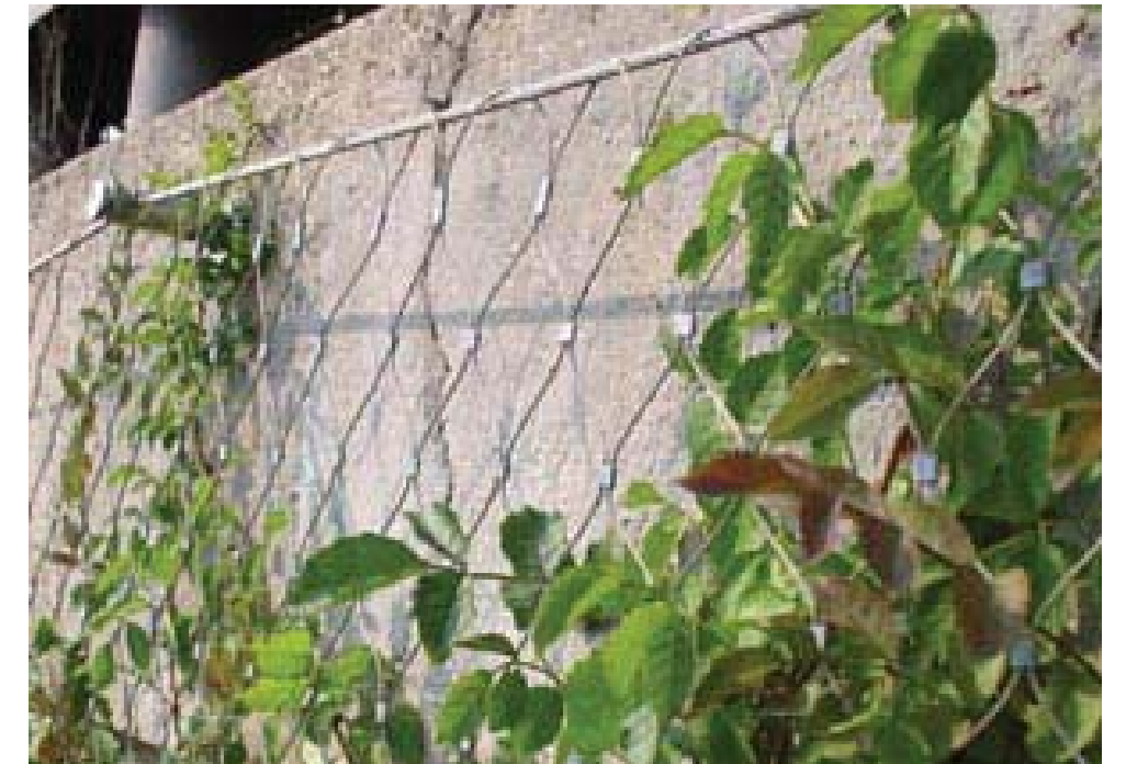
STAINLESS STEEL WIRE MESH AND CABLE TRELLIS
