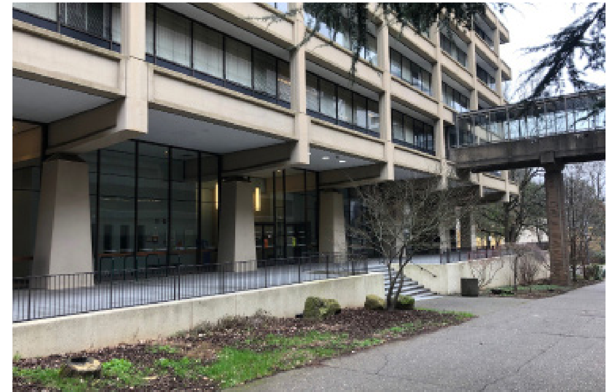
CURRENT APPROACH FROM MILL ST.
