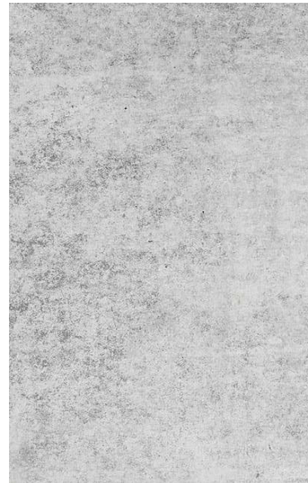
CONCRETE SEAT WALLS (SMOOTH ARCH. FINISH)
