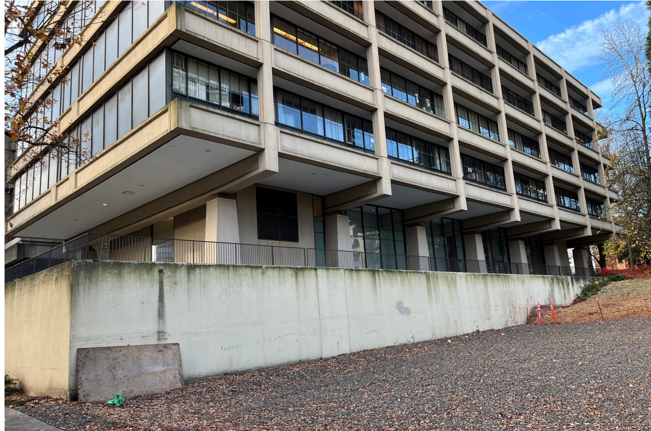
CURRENT NORTH BUILDING EDGE FROM 10TH AVE.
