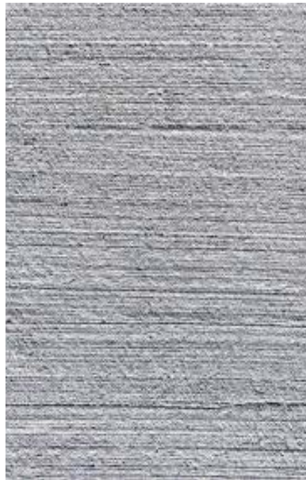
CONCRETE PAVING (MEDIUM BROOM FINISH)
