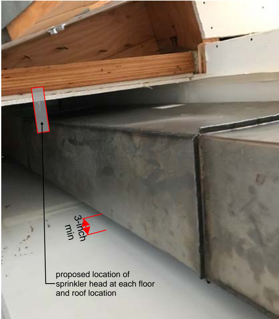
Vent Hood Duct - looking up
