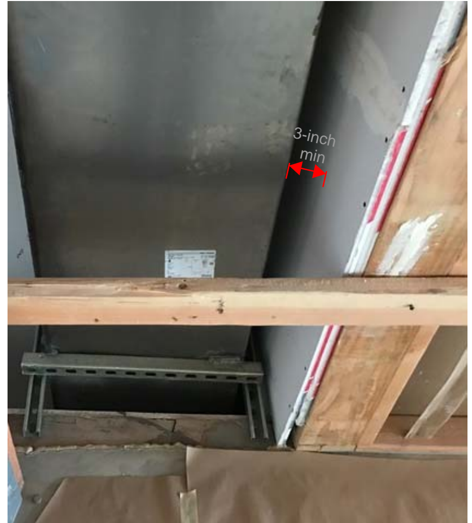
Vent Hood Duct - looking down
