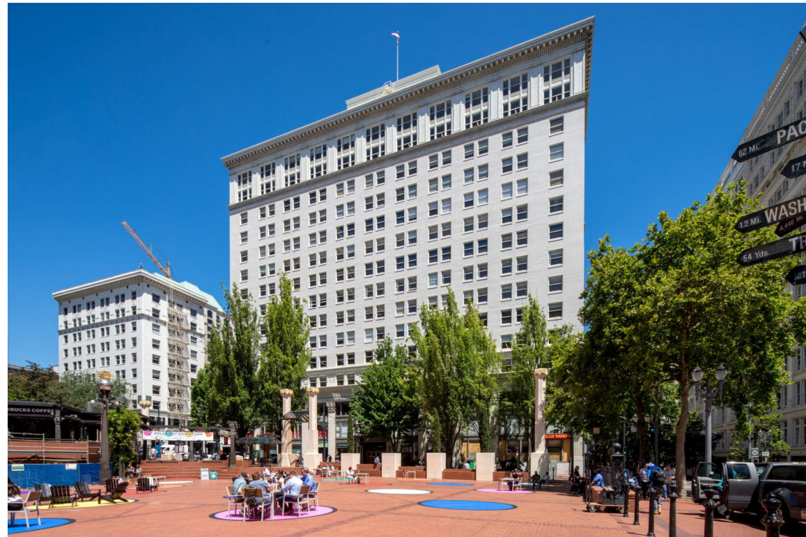
AMERICAN BANK BUILDING
