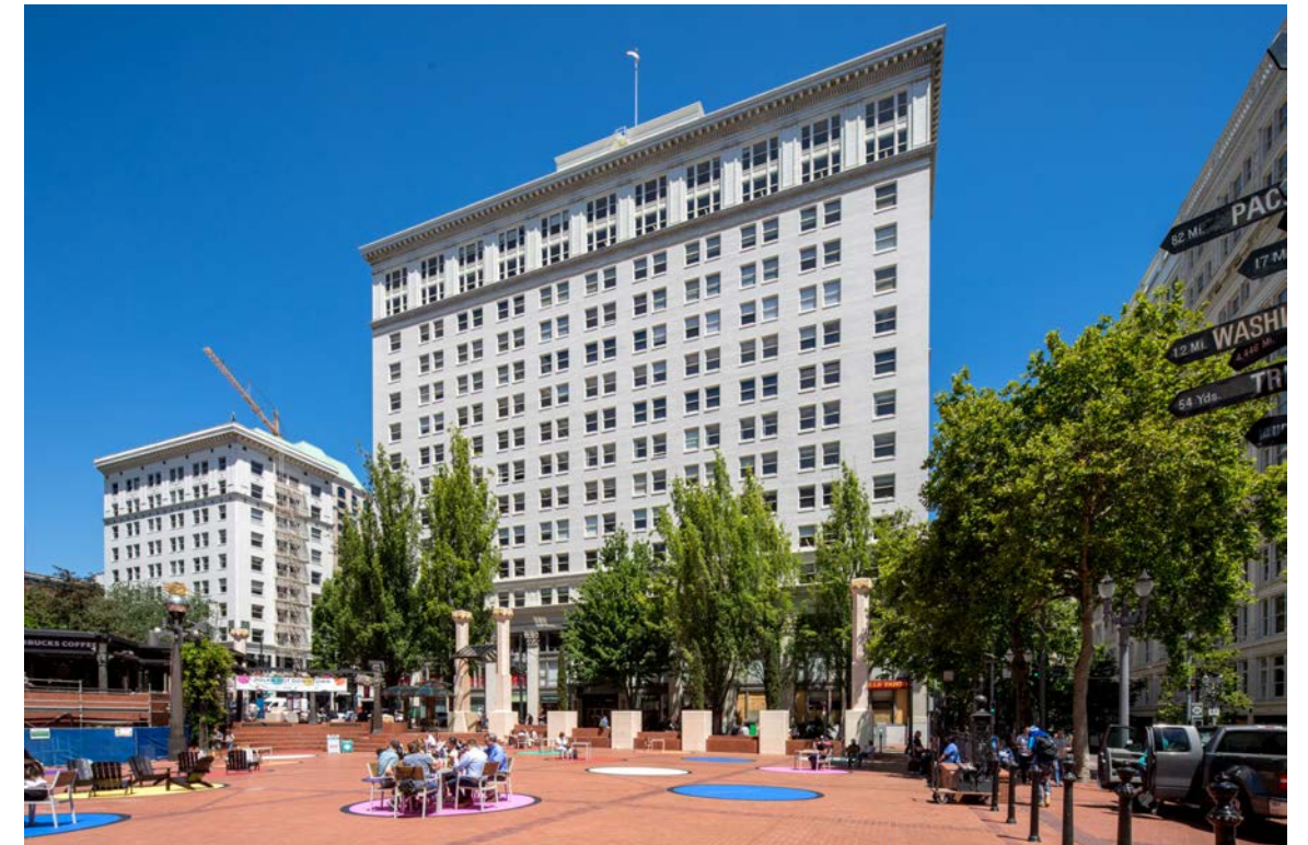
AMERICAN BANK BUILDING
