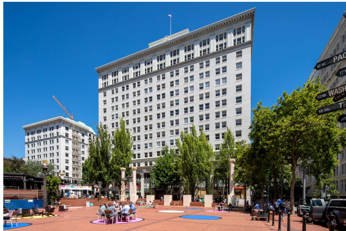
AMERICAN BANK BUILDING
