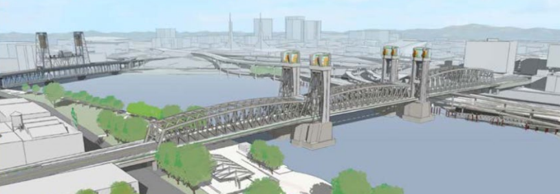
Through Truss Long Span
