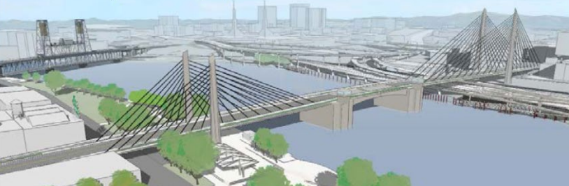
Cable Stayed Long Span
