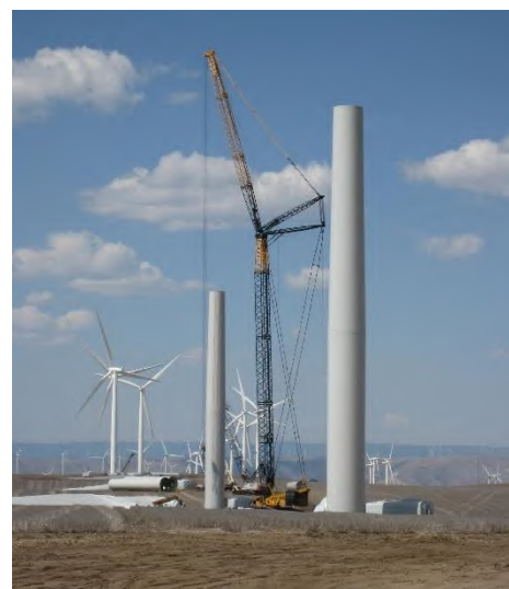
Wind turbine construction in Oregon.
