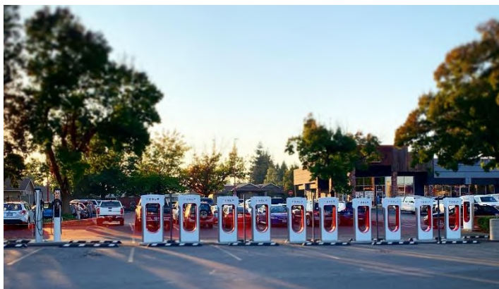
This bank of Tesla chargers was being installed at a northeast Salem shopping center in September 2020.
