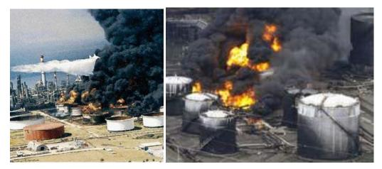
Figure 5: Fire Caused by Tank Damage following 1999 Turkey (left) and 2011 Tohoku Earthquakes (right) (French Ministry of Ecology, Sustainable Development and Energy, 2013)
