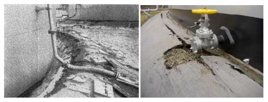
Figure 4: Liquefaction Induced Settlement following 1964 Niigata and 2011 Tohoku Earthquakes in Japan (Watanabe 1966, Zama et al 2012)
