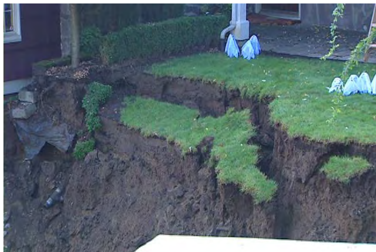
Image: Landslide in Southwest Portland (2008)
