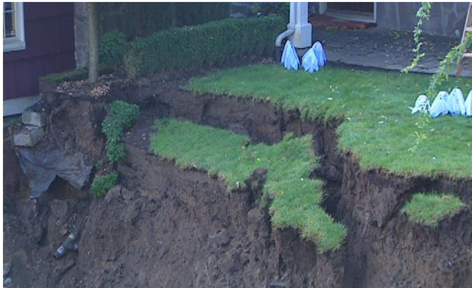
Image: Landslide in Southwest Portland (2008)
