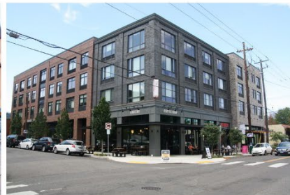
George Besaw Apartments, Portland
