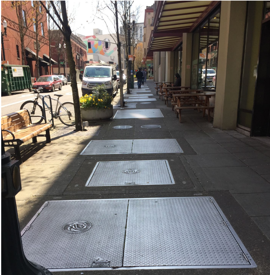
NW 13th between Burnside and Couch
