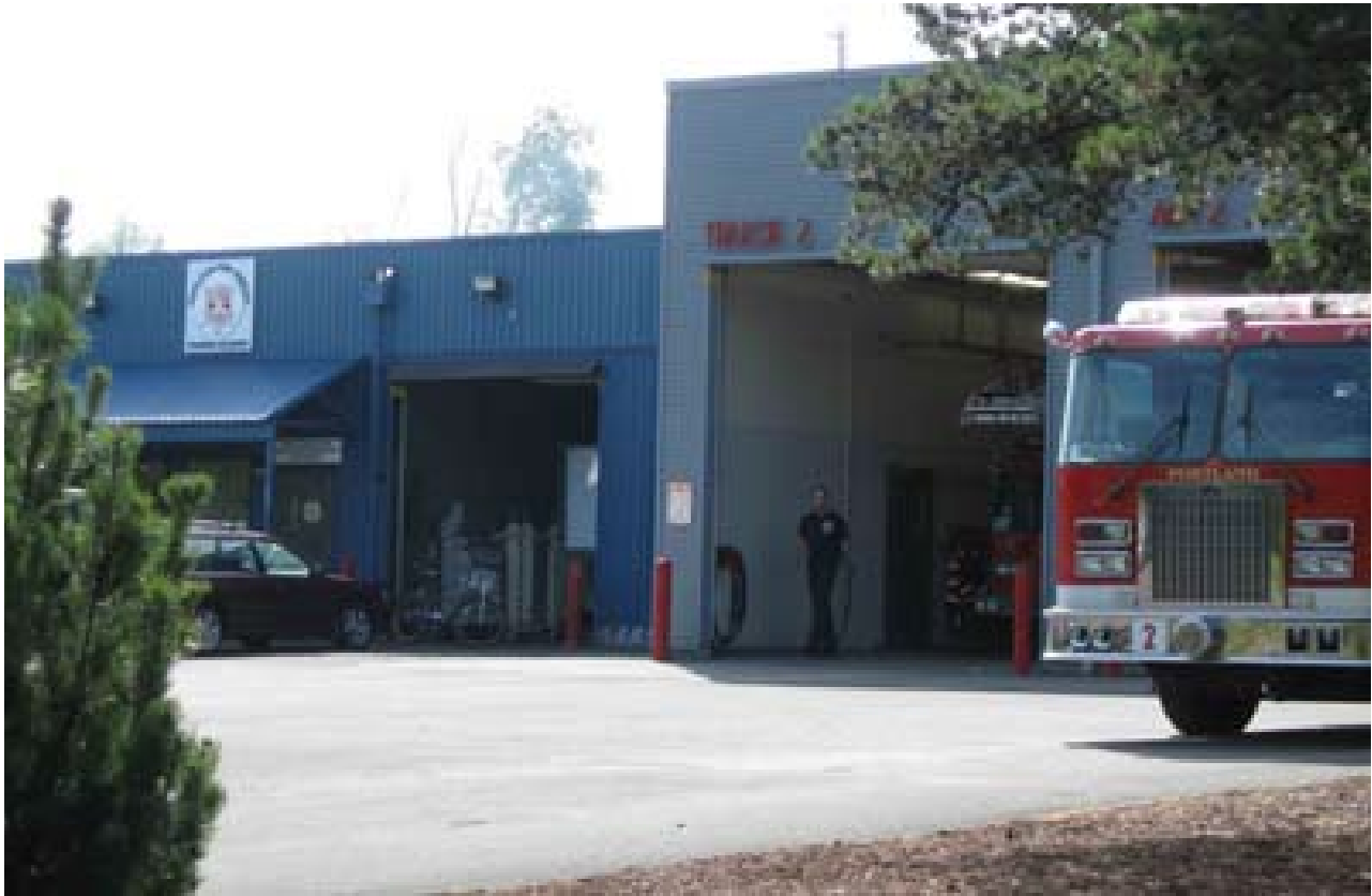
Parkrose Fire Station
