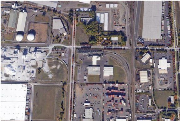
AMD Bulk Terminal (2012-13)
