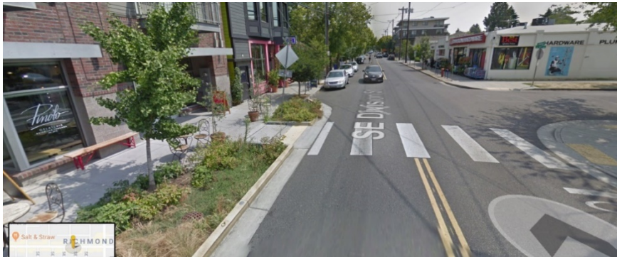
Figure 4-11. Pedestrian Ramp Aligned with the Opposite Corner
