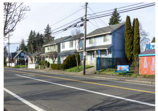
Housing on Flavel Street near 72nd Avenue
