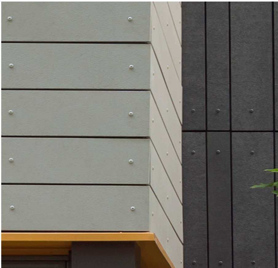
PROJECT: Home Forward Gallagher Plaza, Portland OR, Holst Architecture MATERIAL: Oko Skin Glass Fiber Wall Panel w/exposed screws ENTITLEMENTS: Type III Historic Resource Review
