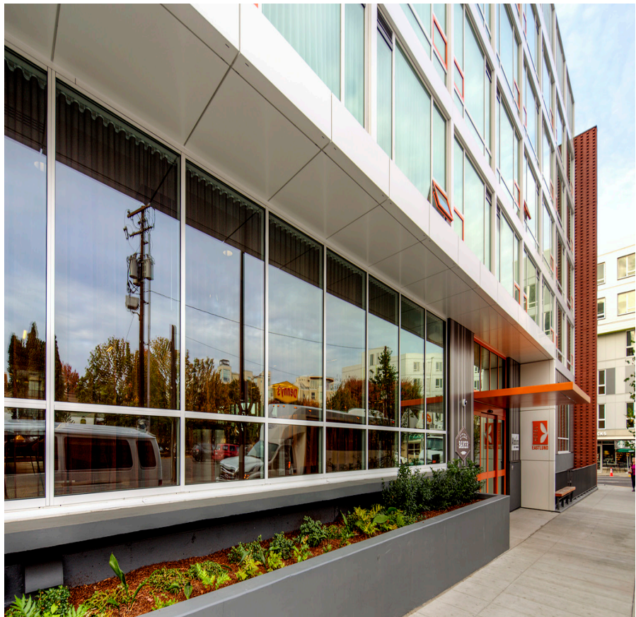
PROJECT: Hotel Eastlund, Holst Architecture MATERIAL: ACM route & return panel w/ concealed attachment
