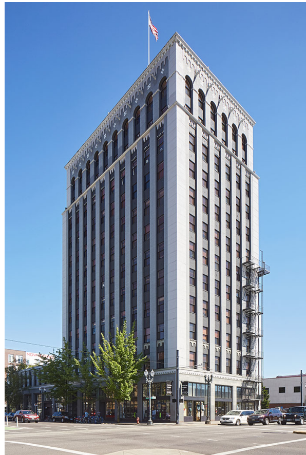
The 1928 Weatherly Building is listed on the National Register and is a contributing building in the East Portland/ Grand Avenue Historic District.
