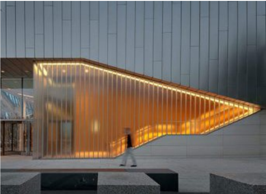
CHANNEL GLASS WALL SYSTEM
