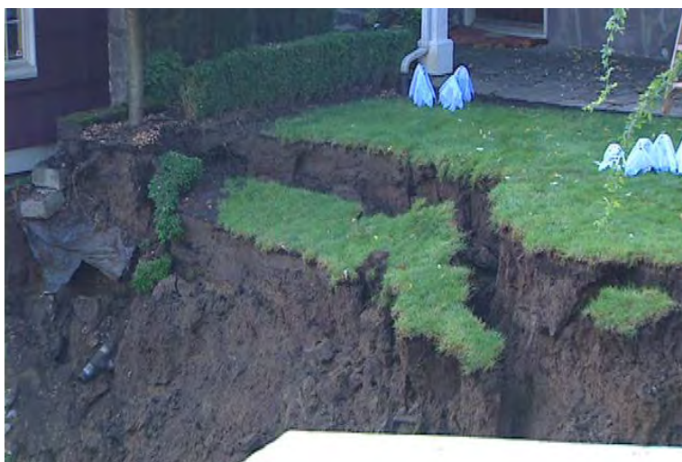
Image: Landslide in Southwest Portland (2008)
