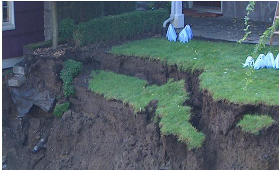
Image: Landslide in Southwest Portland (2008)
