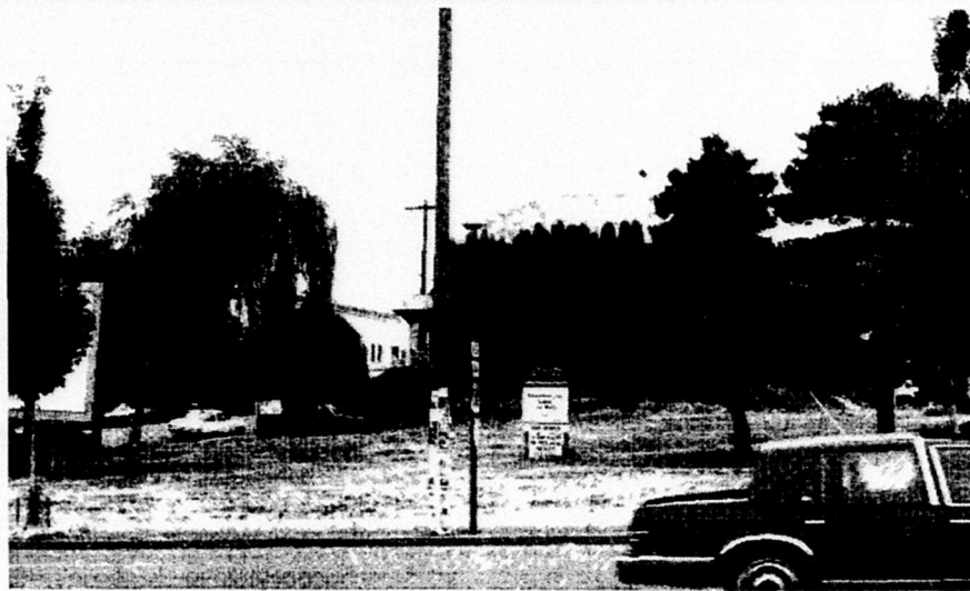
North side of 11th/12th/Burnside
