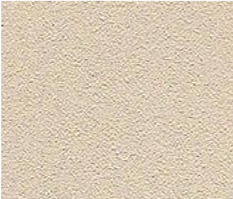
THREE COAT STUCCO, STANDARD FINISH, COLOR TO MATCH METAL PANEL SANDSTONE
