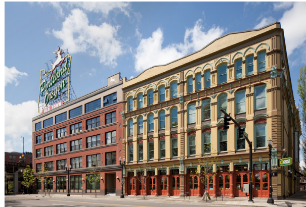
Seismic retrofit of the White Stag Block (bottom) was only feasible due to market-rate tenants and federal/local subsidy programs. Properties such as the Pittock Mansion (top) have a more difficult time funding and accomodating seismic interventions.
