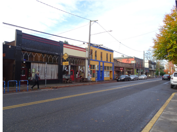
3342 & 3348 SE Belmont proposed for demolition resulting in loss of an intact historic streetscape.
