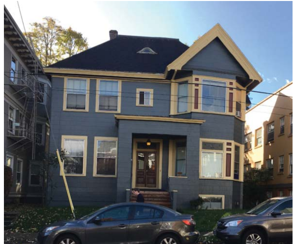
Existing non-contributing 13-unit apartment, slated for demolition
