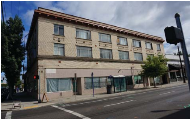
Before Rehabilitation (Exterior)
