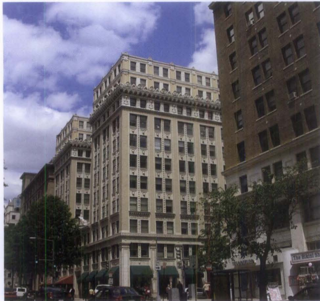
Figure 19. The upper two floors of this early-20th century office building were part of the original design, but were not built. During rehabilitation, the two stories were finally constructed. This treatment does not meet the Standards because the addition has given the building an appearance it never had historically.
