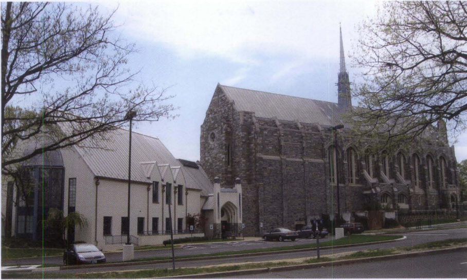
Figure 11. The addition to this early-20th century Gothic Revival-style church provides space for offices, a great hall for gatherings and an accessible entrance (left). The stucco finish, metal roof, narrow gables and the Gothic-arched entrance complement the architecture of the historic church. Placing the addition in back where the ground slopes away ensures that it is subordinate and minimizes its impact on the church (below).
