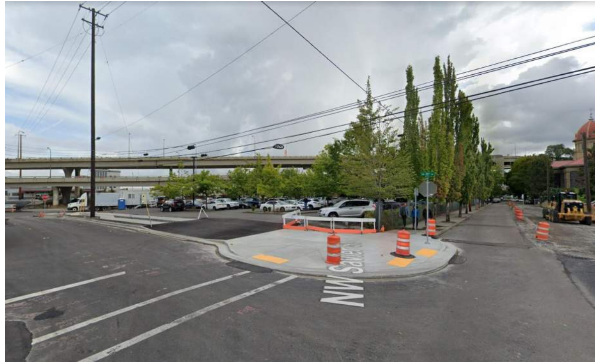
BLOCK 261 FROM SOUTHWEST
