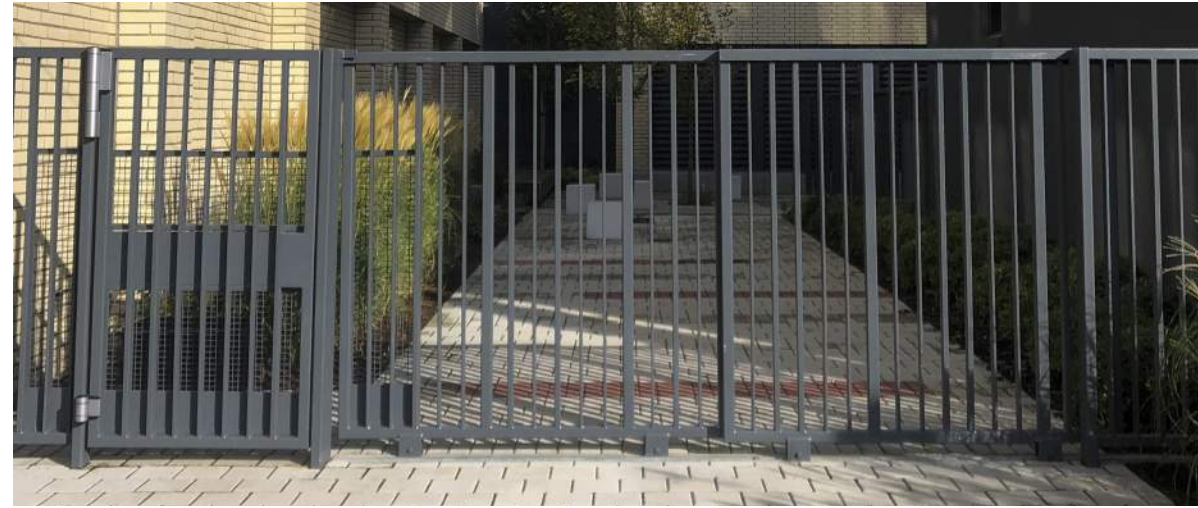
SLIDING GATE WITH MAN DOOR
