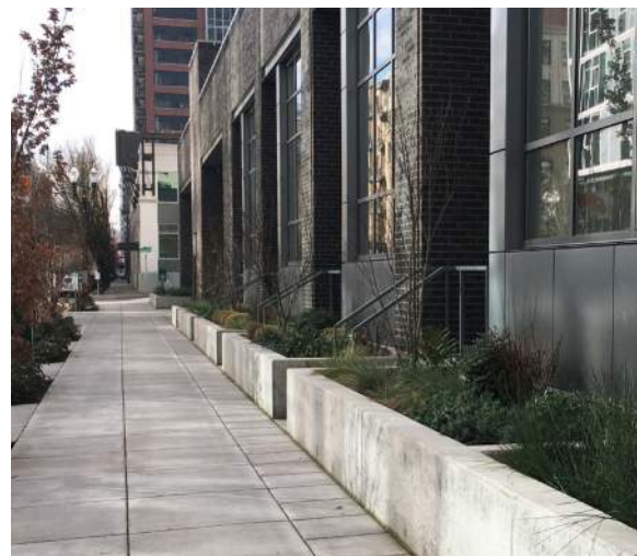
RAISED CONCRETE WALLS AT STOOPS
