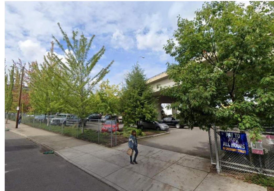
BLOCK 261 FROM SOUTHEAST
