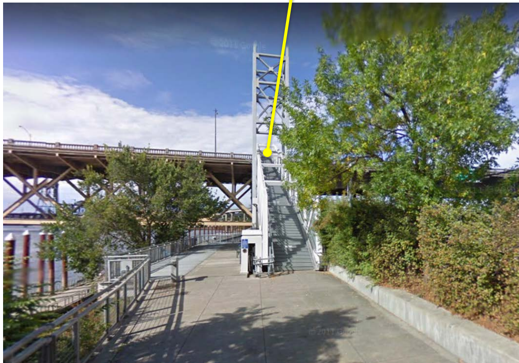
Owner: City of Portland
