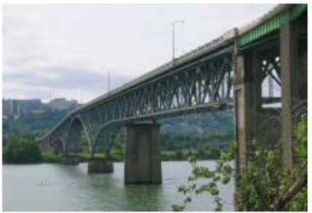
9 Ross Island Bridge
