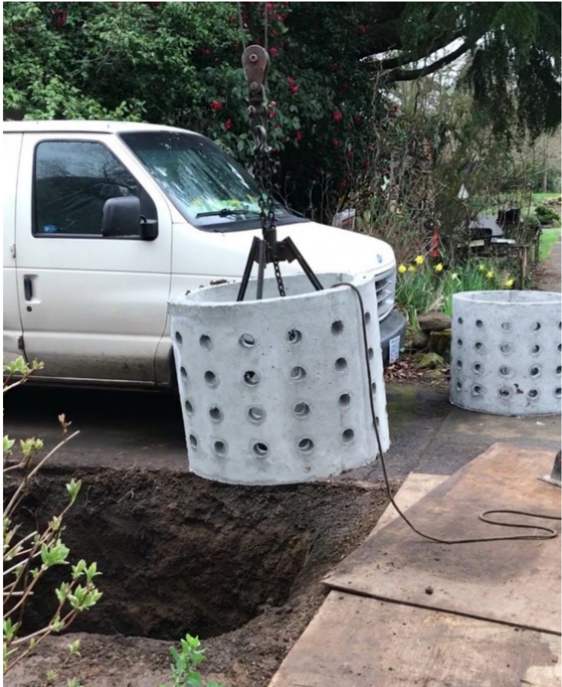
Figure 17 Example retrofit #2, SE Richmond 28" x 5' drywell installation
