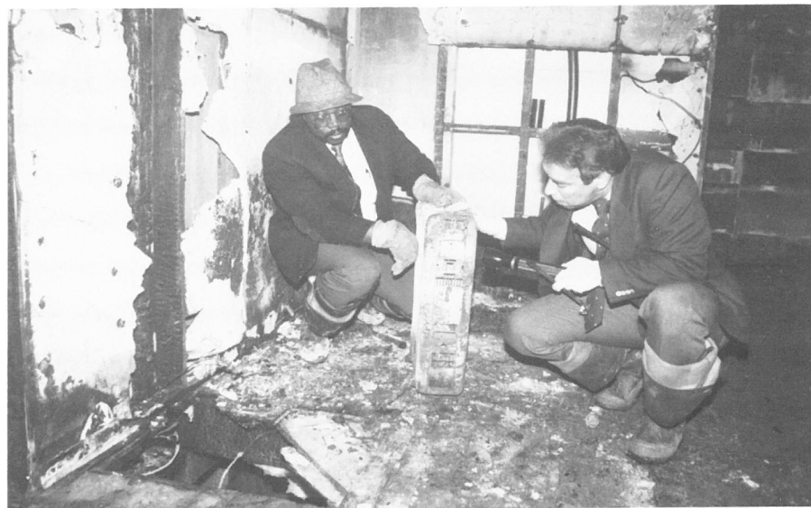
Fire Investigators checking possible source of ignition.
