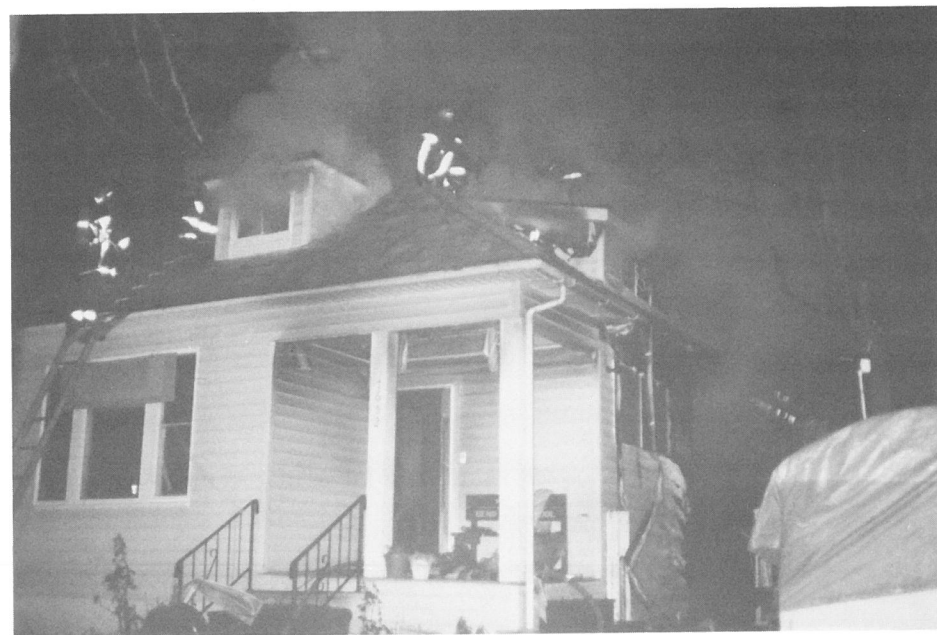
Two story house fire igniting in the basement and spreading to the second floor
