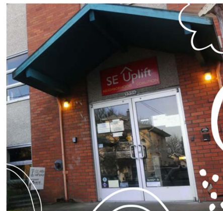
Figure 13. SEUL Main St. Office
