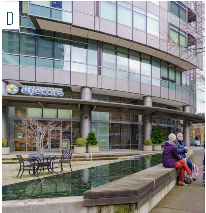
Incorporating stormwater into the design of open areas. This stormwater system uses the grade change to provide a seat wall amenity. South Waterfront, SW Gaines and SW River Parkway
