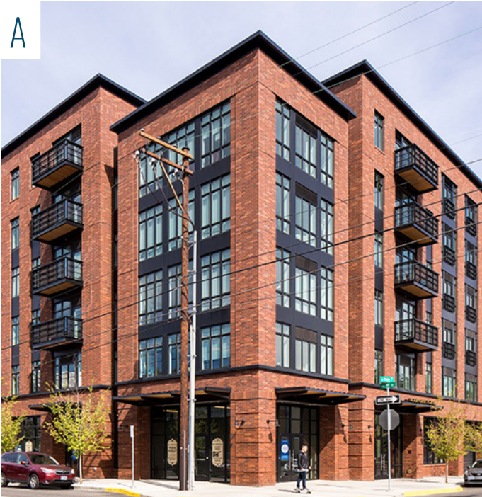
Emphasizing the corner through massing shifts. This corner site offers an opportunity to provide a prominent entry and upper level terrace. Northwest District, NW 19th and NW Quimby
