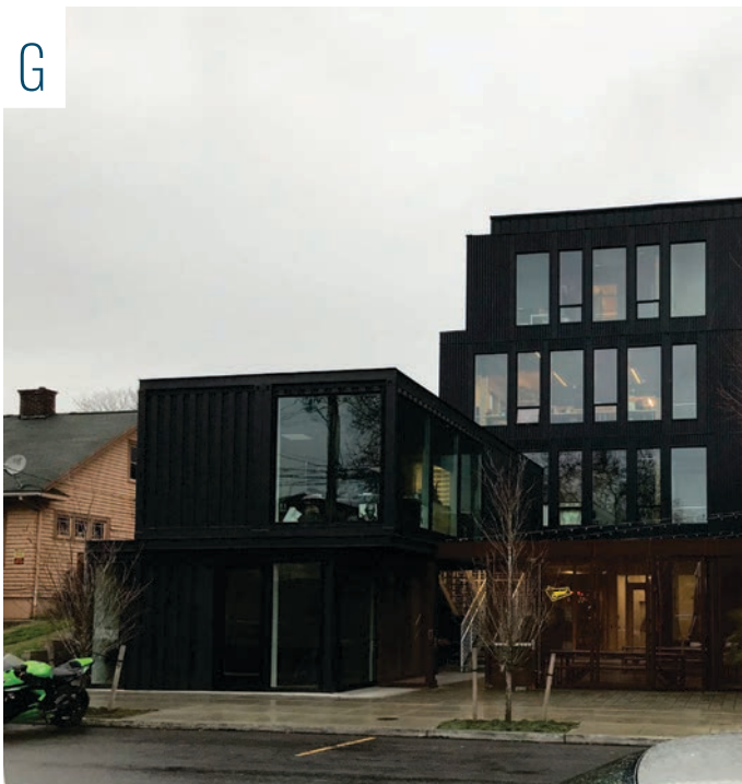
Breaking up building massing where it is adjacent to lower density residential to reduce the contrast between scales in height. Mississippi, N Albina and N Blandena
