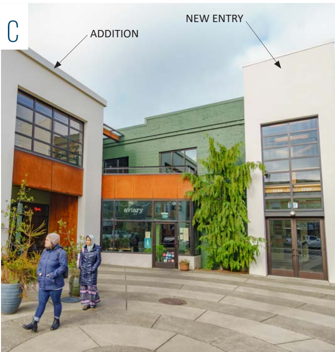
Creating an addition that references existing architecture. This addition integrates similar materials in its new entry and the new building and connects both with special paving and a shared courtyard. Alberta, NE Alberta and NE 18th
