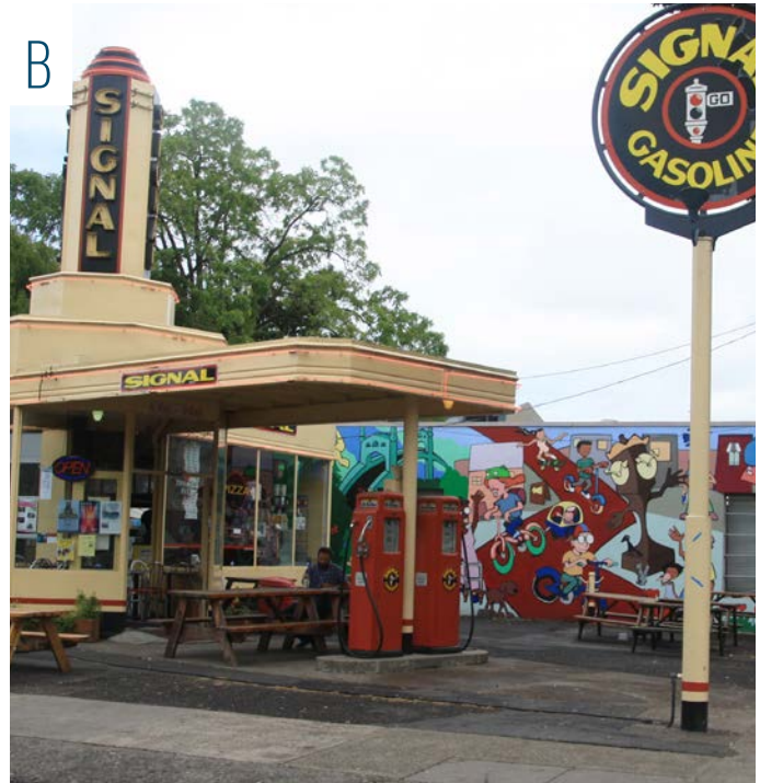
Maintaining a site's uniqueness by re-purposing architectural elements, such as sculptural neon signage and character defining canopies. St. Johns, N Lombard and N Charleston
