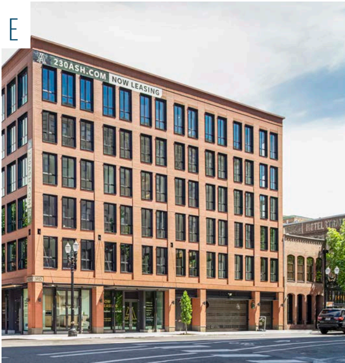
Aligning belt courses and window heights. This newer building on the left uses the same vocabulary as its historic neighbor: materials, repetition of bays and windows, and continuity of setbacks. Old Town/Chinatown, SW 3rd and SW Ash
