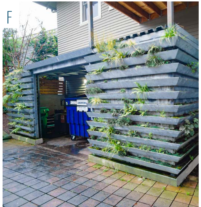
Tucking and screening waste bins. This trash and recycling area is well-hidden from the building's street-facing façade and artfully screened behind a planter designed to capture rainwater. Division, SE Division and SE 38th
