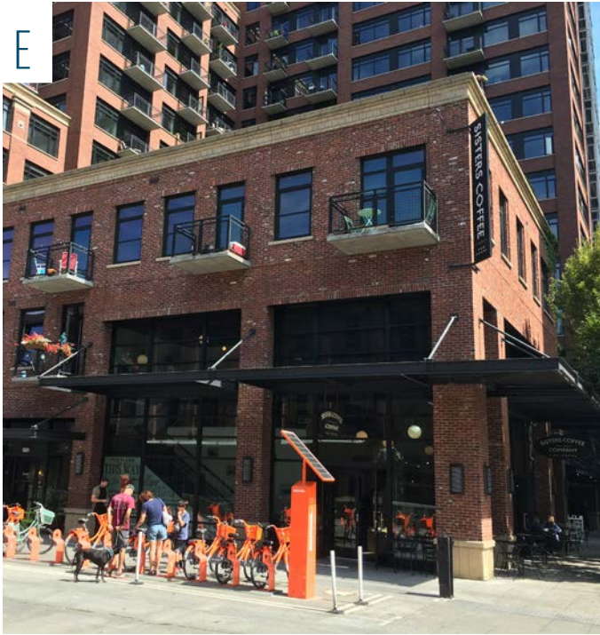
Reusing salvaged brick in the façade of new buildings. This example references its site's history and conserving valuable resources. Pearl, NW Marshall and NW 13th
