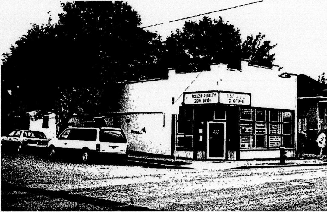
This storefront on 52nd Avenue is an example of Streetcar Era Commercial style
