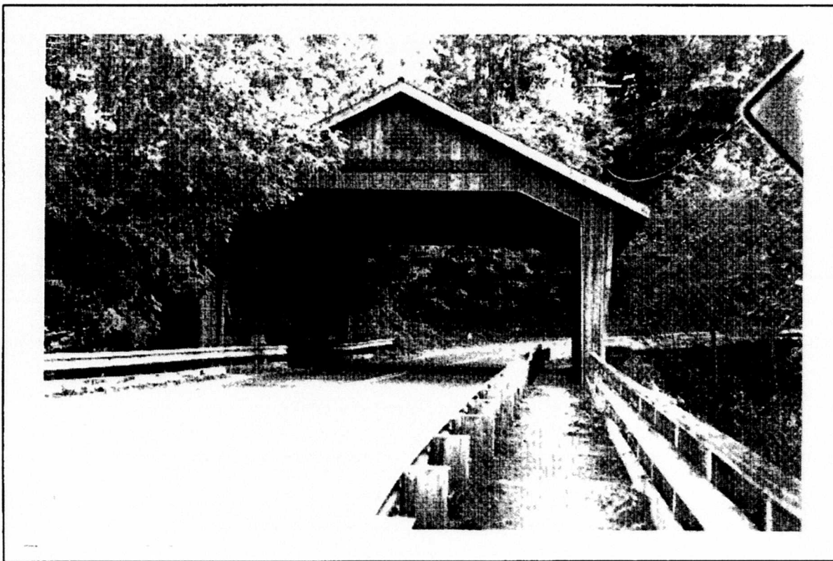
Cedar Crossing Bridge Johnson Creek and Deardorff Road
