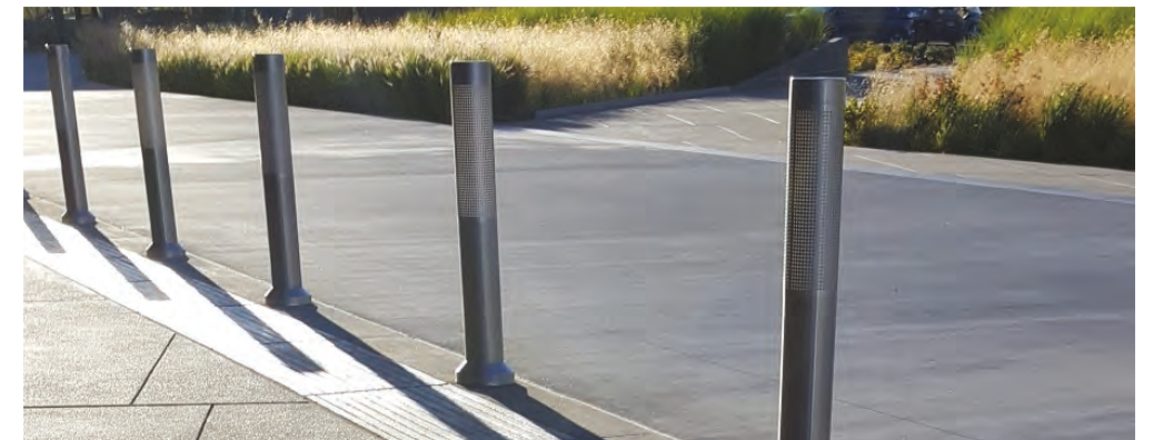
Example of bollards proposed along path opposite Portland Art Museum (Daimler headquarters, Mayer/Reed)
