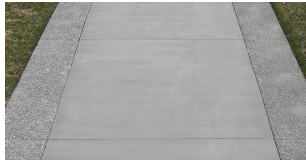
Paving Option 2 (for full block rehabilitation): Single pour, cast-in-place 6" reinforced concrete panels with broom finish and exposed aggregate edge accent (or vice versa). For more contrast to existing paving, use above left.
