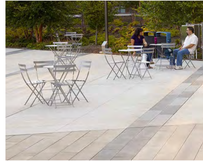
Cast-in-place reinforced concrete with scoring pattern, accent banding, and layout to reinforce pedestrian scale, artwork, and existing and proposed site furnishings (Marion Brenner)
