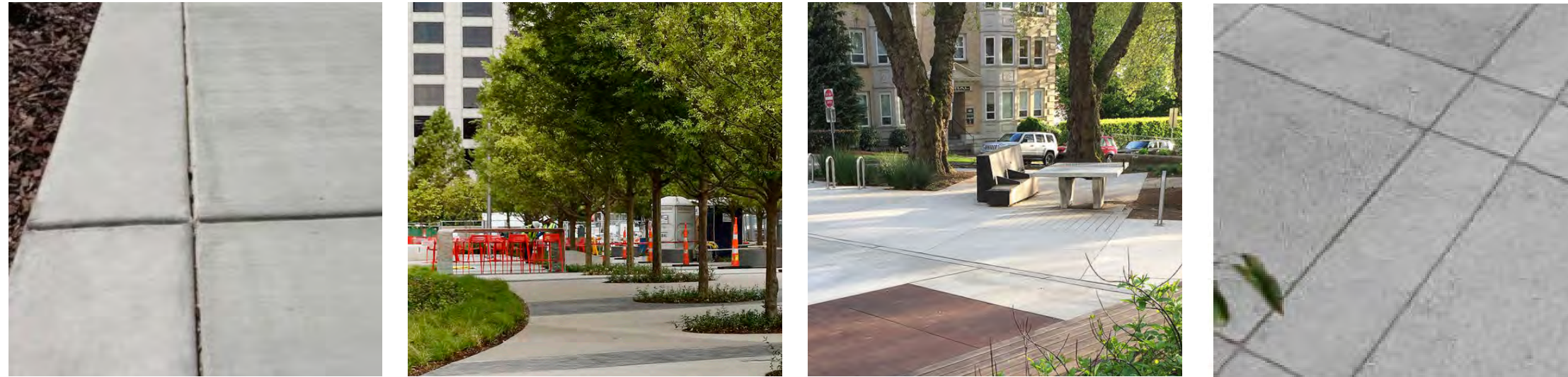
Cast-in-place 6" reinforced concrete, scoring pattern, tooling, accent curb headers, slip resistant finish. New concrete will darken over time from exposure to weather and urban conditions so it visually fades back.
