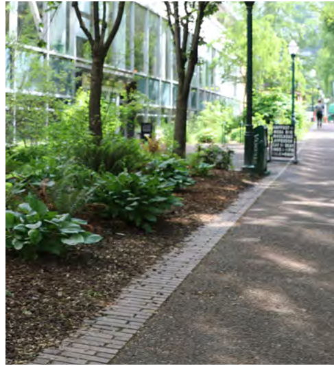
Paving Option 1 (for small repairs prior to full block rehabilitation): Match existing exposed aggregate paving with brick border. Finish of new pavement to match adjacent paving while meeting ADA thresholds.
