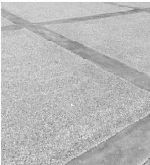
Paving Option 2 (for full block rehabilitation): Single pour, cast-in-place 6" reinforced concrete panels with broom finish and exposed aggregate edge accent (or vice versa). For more contrast to existing paving, use above left.
