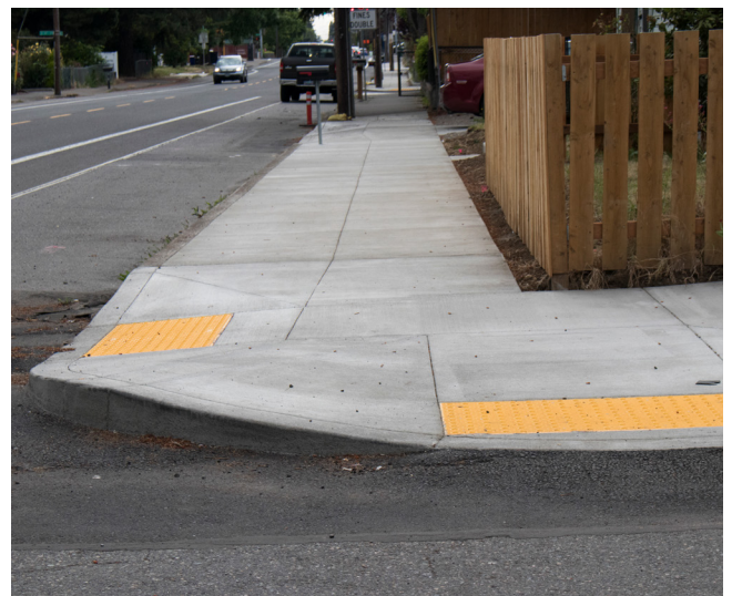
Recently installed curb ramps in Portland.
