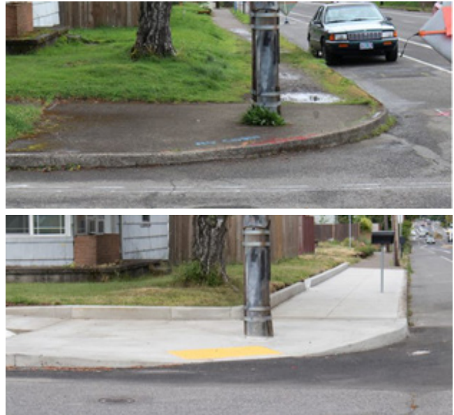
A before and after photo of curb ramp in Portland.
