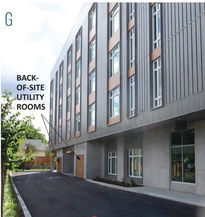
Placing mechanical and utility rooms away from the street-facing facades and providing well-integrated screening. Gateway, SE 105th and E Burnside
