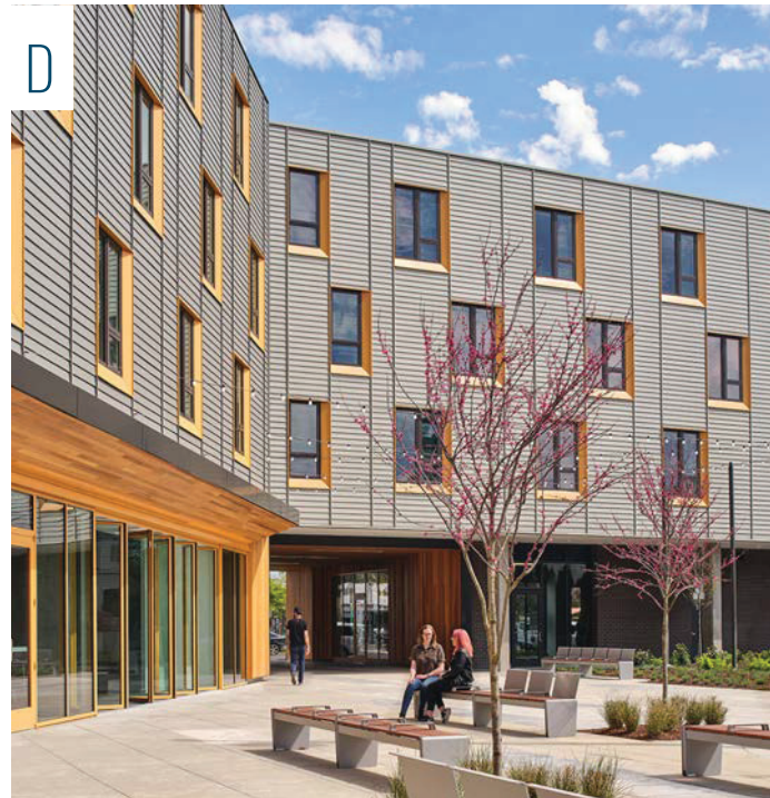
Expressing building function and hierarchy by emphasizing the ground floor with high quality materials and using repetition in the design and placement of upper level openings and materials. Heart of Foster , SE Foster and SE 72nd
