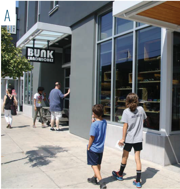
Designing covered entries, signage, seating, and glazing details that contribute to interest and activity at the human-scale. Alberta, NE Alberta and NE 21st
