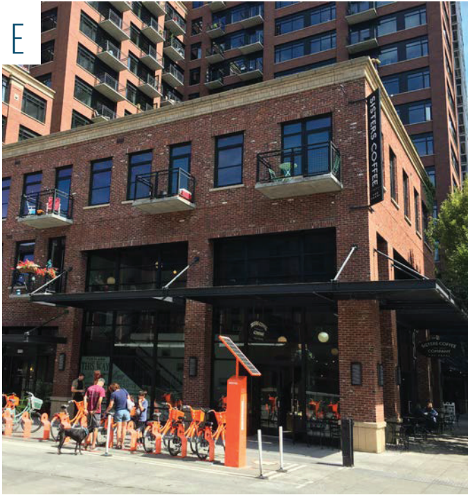
Reusing salvaged brick in the façade of new buildings. This example references its site's history and conserving valuable resources. Pearl , NW Marshall and NW 13th
