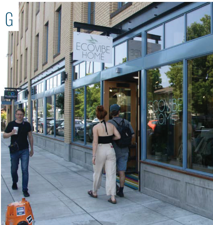
Drawing on traditional materials and patterning to create an organized and articulated ground floor. Heavy masonry materials, such as brick and concrete extend to the ground to express the building's structure. Alberta, NE Alberta and NE 19th
