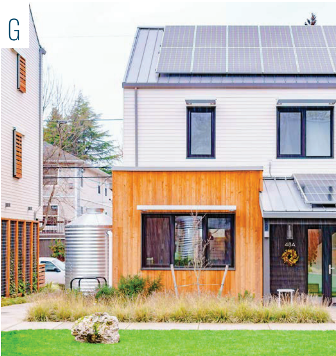
Striving towards net zero with features that include photovoltaic panels on all south-facing roofs, triple-paned windows to limit the amount of hot and cold air and cisterns for collecting rainwater. Eliot , NE Williams and NE Tillamook
