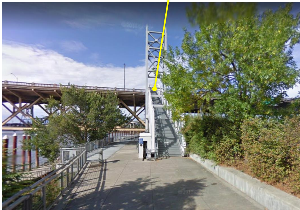
Owner: City of Portland
